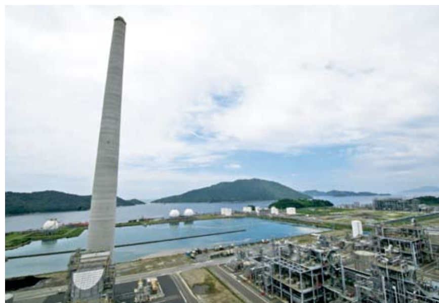
A host of systems for removing dust and pollutants from plant exhaust help minimize the environmental impact of Tosoh's manufacturing operations.
