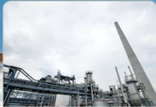
A doubling of production capacity for aniline was part of a recent expansion of the vinyl isocyanate chain operations at Tosoh's Nanyo Complex.
