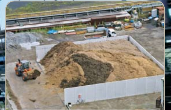
Brown biomass shares the fuel yard with coal alongside the electric power plant at Tosoh's Nanyo Complex—part of the company's efforts to reduce reliance on fossil fuels.
